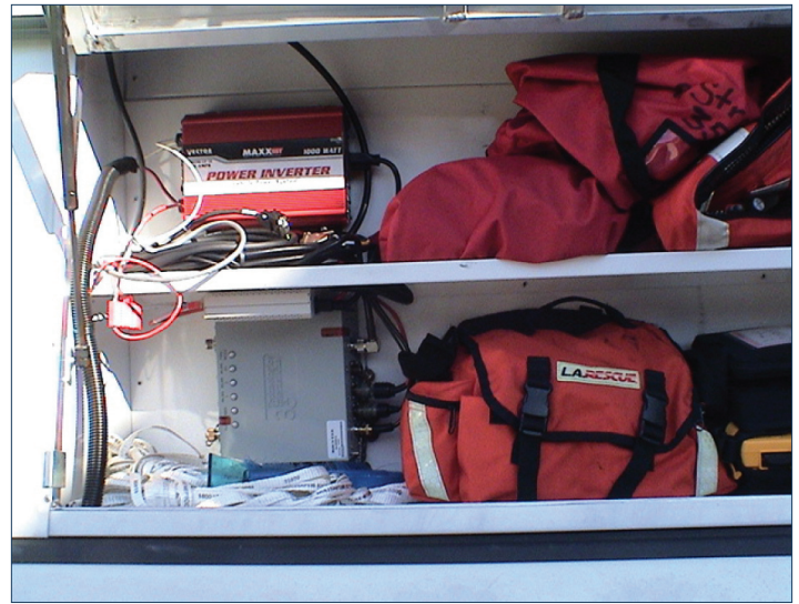
3e-525V-3 video server (mounted on the bottom shelf)
